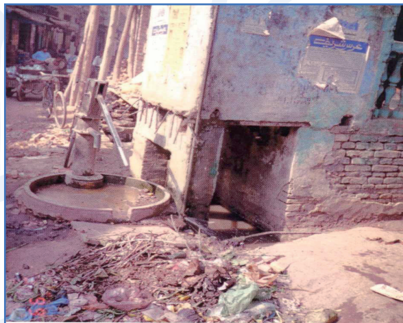
Figure 8: Water contamination due to the unhygienic location
