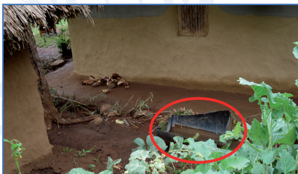
Figure 5: Rainwater harvesting container below the roof of a house Source: Sophia Githinji
